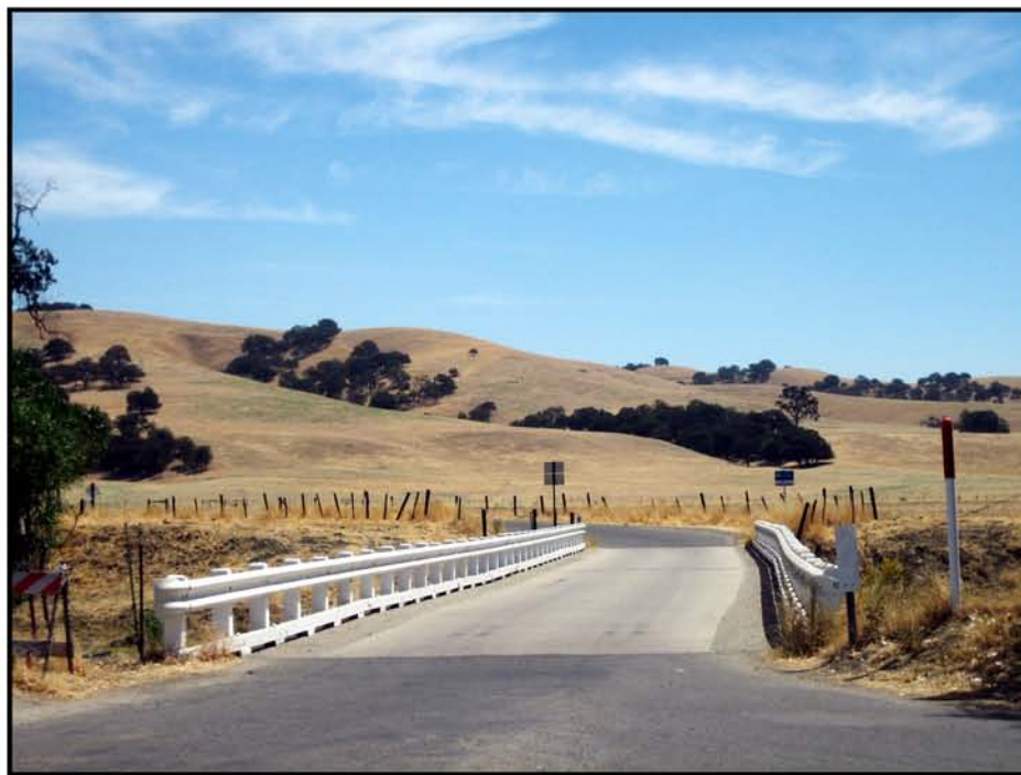
Parkfield Bridge, the San Andreas Fault runs directly underneath.
